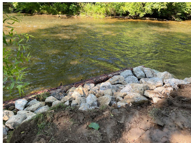
Figure 29: Example of a fortified bank with rip-rap.
