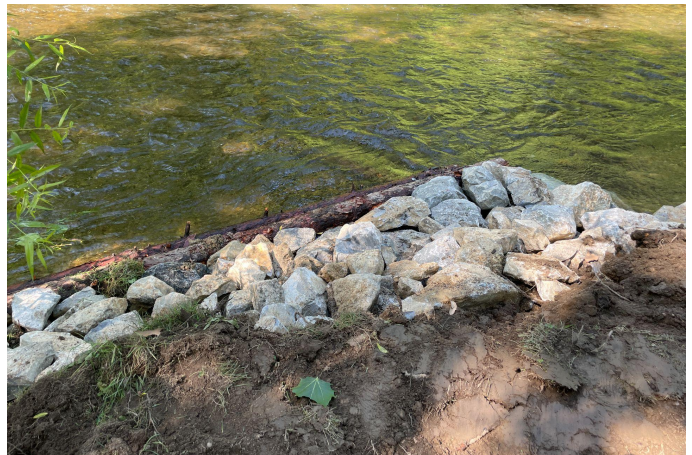
Figure 31. Example of a fortified bank with rip-rap. Photo credit: ALLARM
